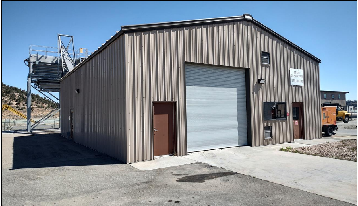
Solid separation Building
