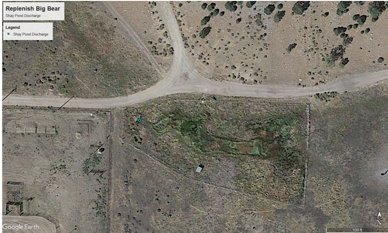
Figure 12. Shay Pond Aerial View
