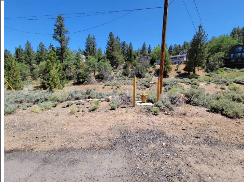
Photo 23. Potential Sand Canyon Recharge conveyance pipeline discharge outlet to Sand Canyon location (2022).
