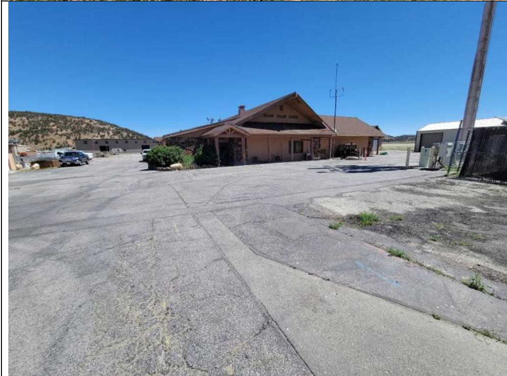
Photo 16. BBARWA WWTP Upgrades site (2022).
