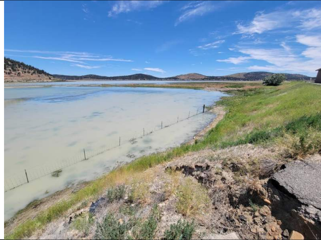
Photo 13. East end of proposed new solar evaporation ponds site, looking northeast (2023).
