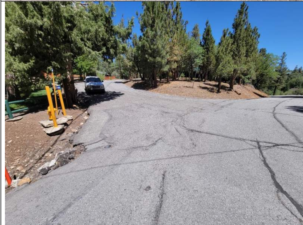
Photo 22. Representative Sand Canyon Recharge conveyance pipeline alignment in Moonridge neighborhood (2022).
