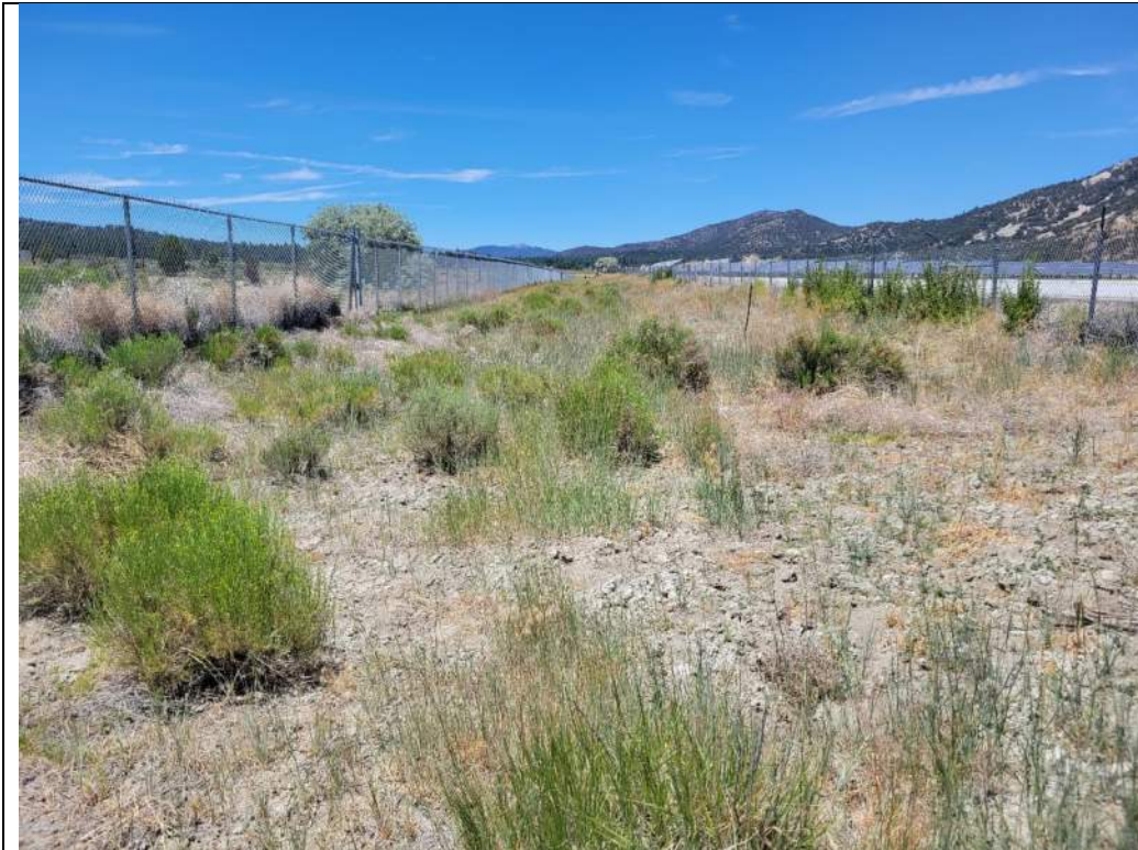
Photo 5. Baldwin Lake conveyance pipeline alternative; looking west along alignment from the east end of the alignment within the BBARWA WWTP (2023).
