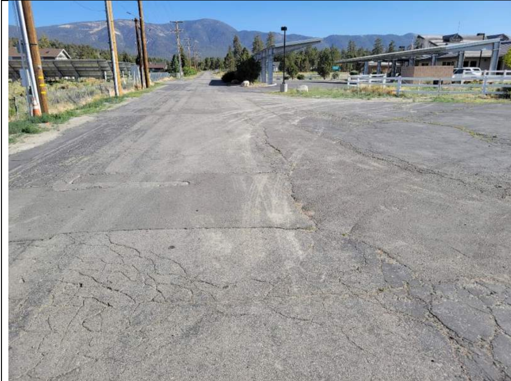
Photo 1. East Neighborhoods conveyance pipeline alternative; looking south along Palomino Drive from the BBARWA WWTP (2022).
