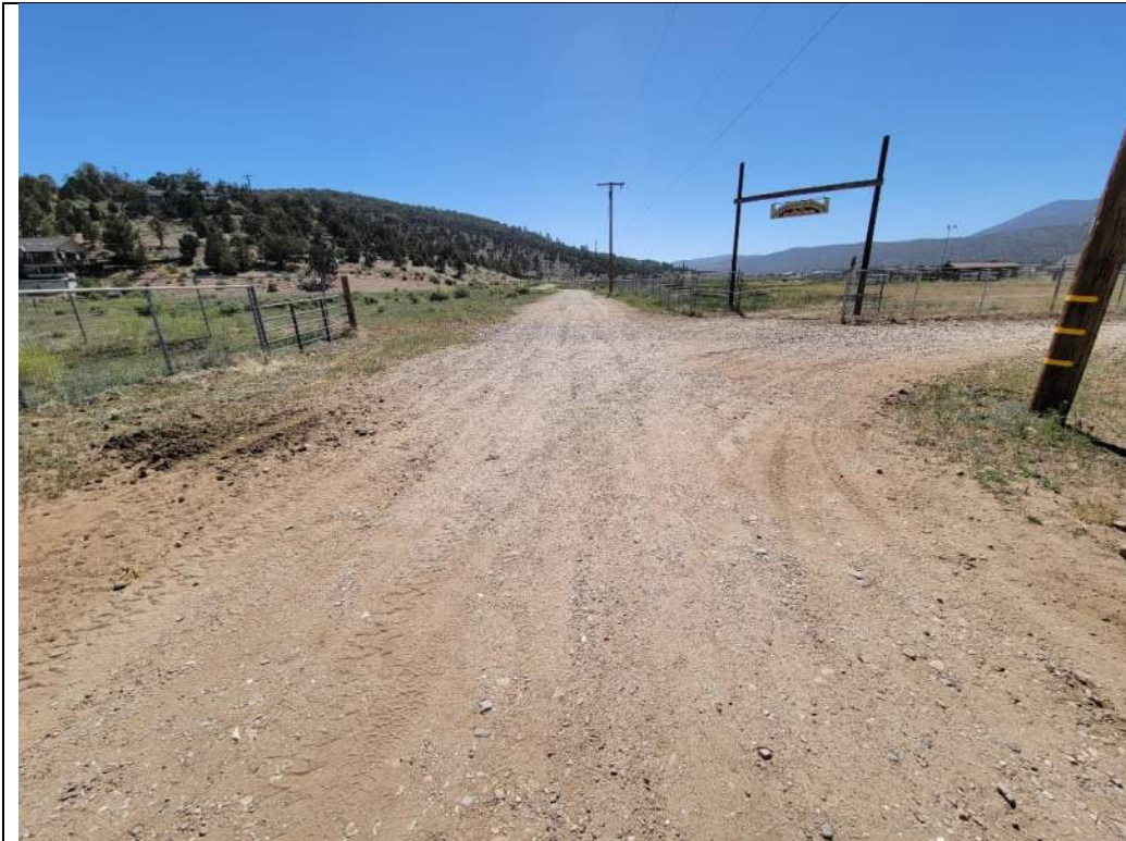
Photo 19. New 4-inch Shay Pond conveyance pipeline alignment in Cascade Street; looking east from west end of alignment (2022).
