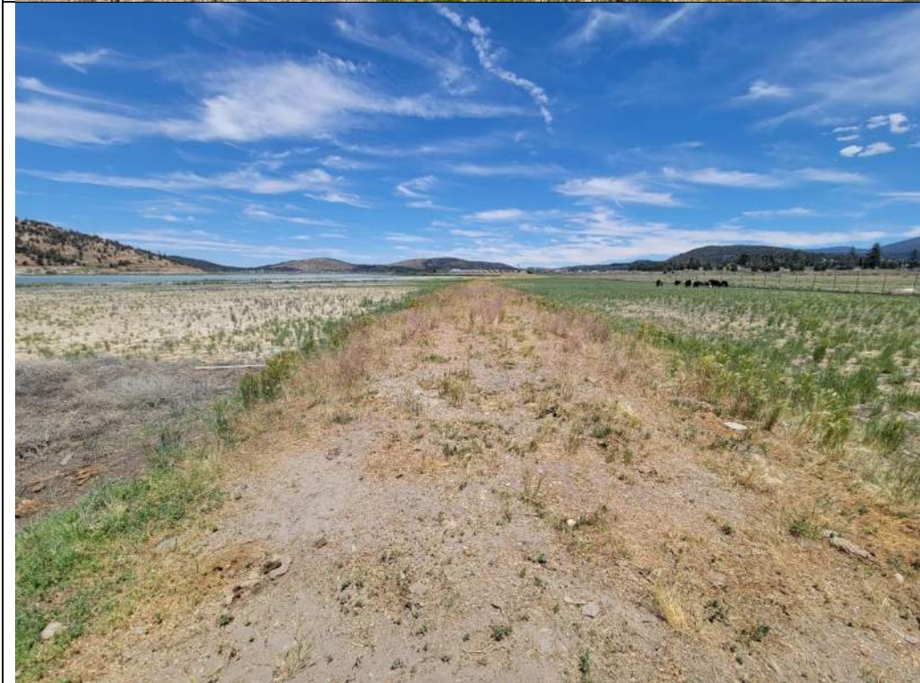
Photo 6. Baldwin Lake conveyance pipeline alternative; looking west along alignment from the east end of the alignment within the W Baldwin Lake Trail (2023).
