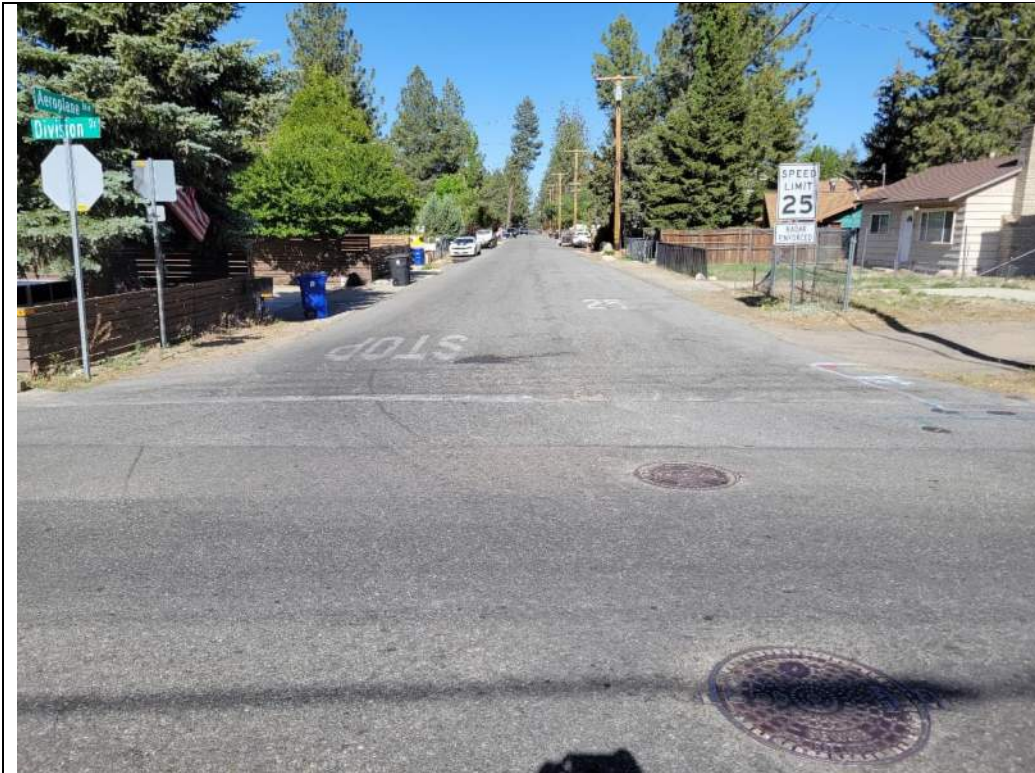
Photo 3. Representative photo of the West Neighborhoods conveyance pipeline alternative; looking east along Aeroplane Boulevard from the intersection of Aeroplane Boulevard and Division Drive (2022).
