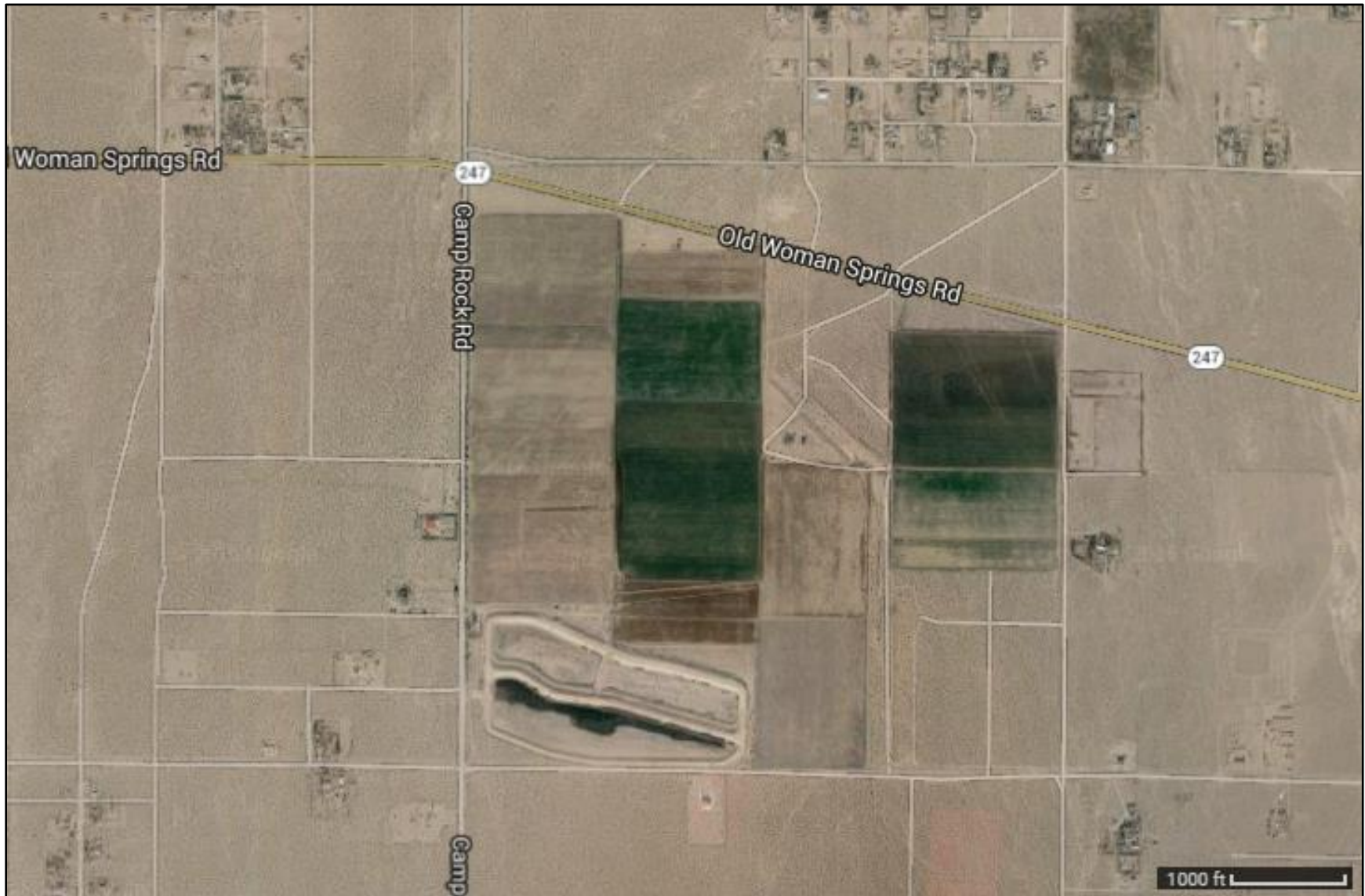
BIG BEAR AREA REGIONAL WASTEWATER AGENCY, OWNER/OPERATOR EXPORT OF RECYCLED WATER TO LUCERNE VALLEY Lucerne Valley – San Bernardino County
